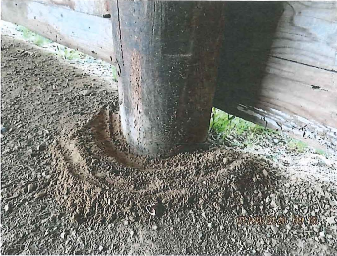
Photograph 13 Minimal Amount of Deterioration at Base of Wood Post
