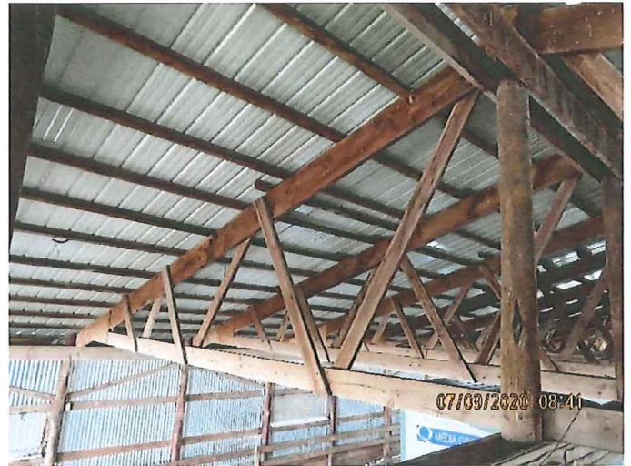
Photograph 6 Roof Truss Wood Framing
