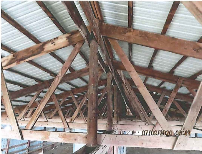
Photograph 5 Two Halves of Roof Truss Meet at Center Posts
