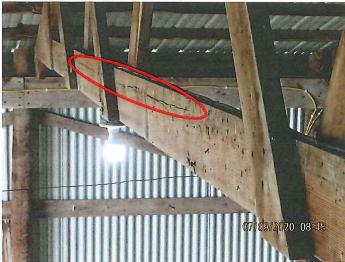
Photograph 11 Check Within Bottom Chord
