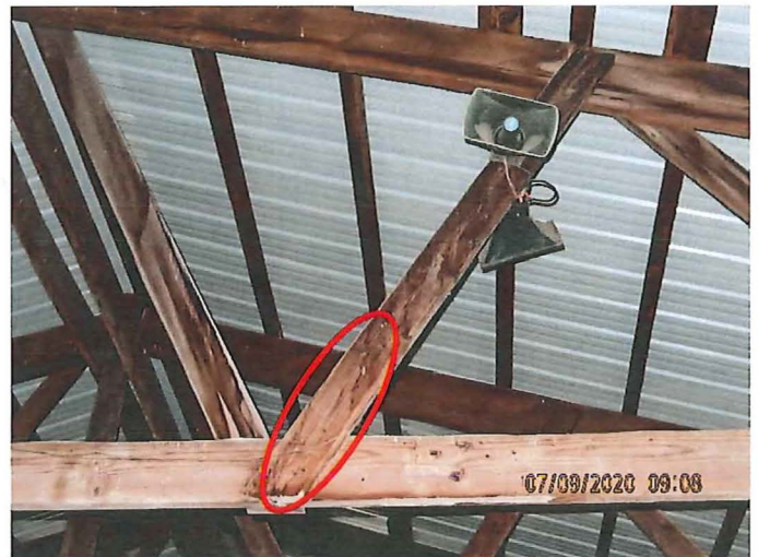
Photograph 8 Ruptured Diagonal Framing Member
