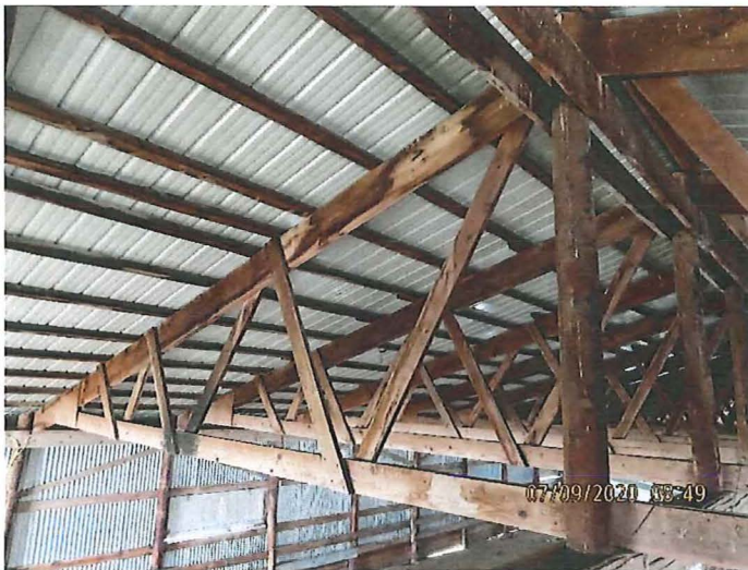
Photograph 7 Water Staining Throughout Framing Members
