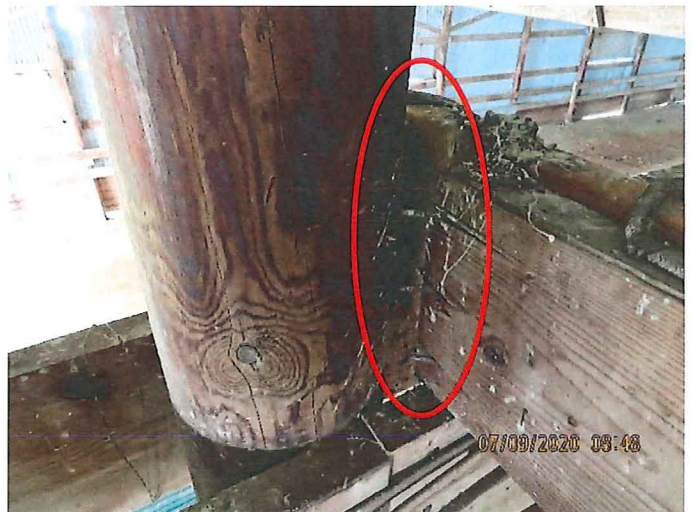
Photograph 20 Deformation and Disengagement of ( End Condition #15 )
