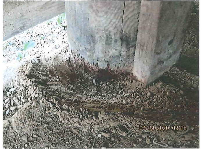
Photograph 14 Wood Decay at Base of Wood Post ( End Condition #15 )
