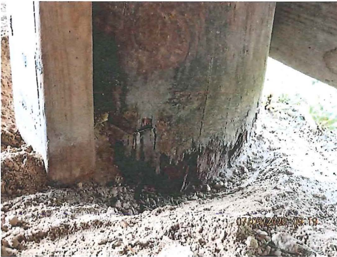
Photograph 15 Wood Decay at Base of Wood Post ( End Condition #15 )
