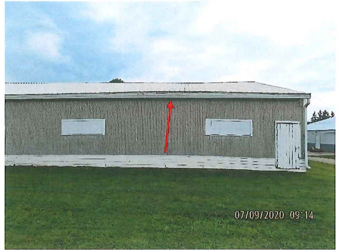
Photograph 10 Upward Displacement Along East Wall Elevation
