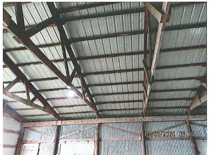
Photograph 4 Wood Posts and Framing at West Wall Elevation
