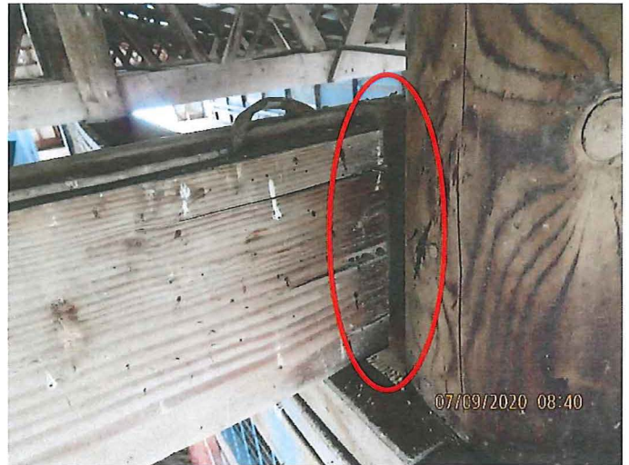
Photograph 18 Detached Bottom Chord Framing Element
