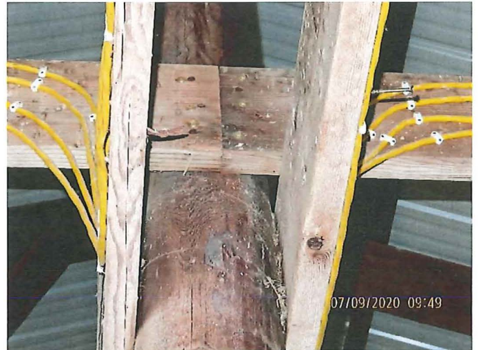
Photograph 16 Bottom Chord at Center Post ( End Condition #2 )
