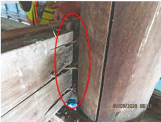
Photograph 19 Deformation and Disengagement of ( End Condition #15 )
