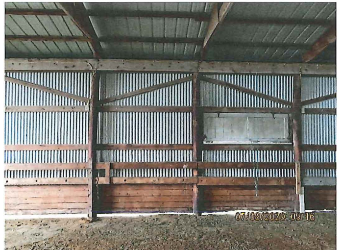
Photograph 12 Displaced Wood Posts Along East Wall Elevation
